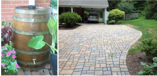
A rain barrel (above left) and permeable pavement (above right)
